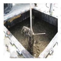
Pictured to the left is an Anoxic Mixer at a WWTP in Florida. The hydrofoil impellers installed here bind up with rags and other fibrous materials until the blades, shaft or mixer drive require maintenance and/or replacement.
